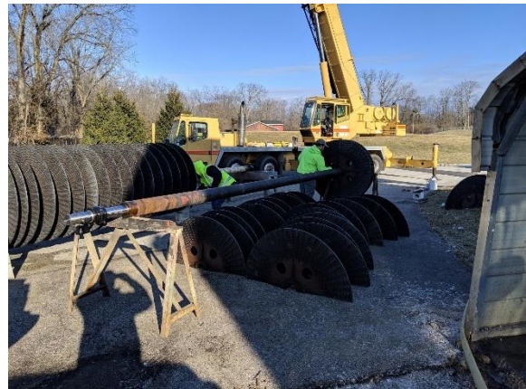
Repairs being made at the Wastewater Treatment Plant
